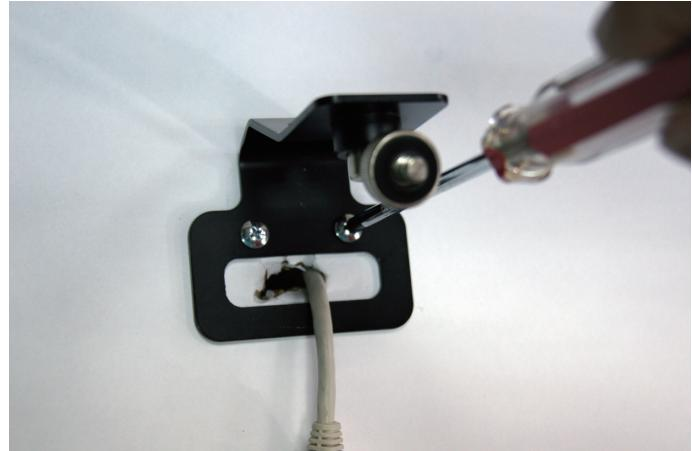
**2. First, pass the network cable through the hole of the stand, then fasten the screws with stand into the wall.**
